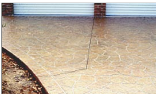
Figure 3: Joint perpendicular to slab edge
